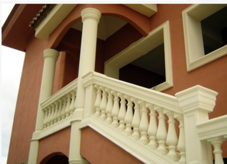
balastra in cemento
